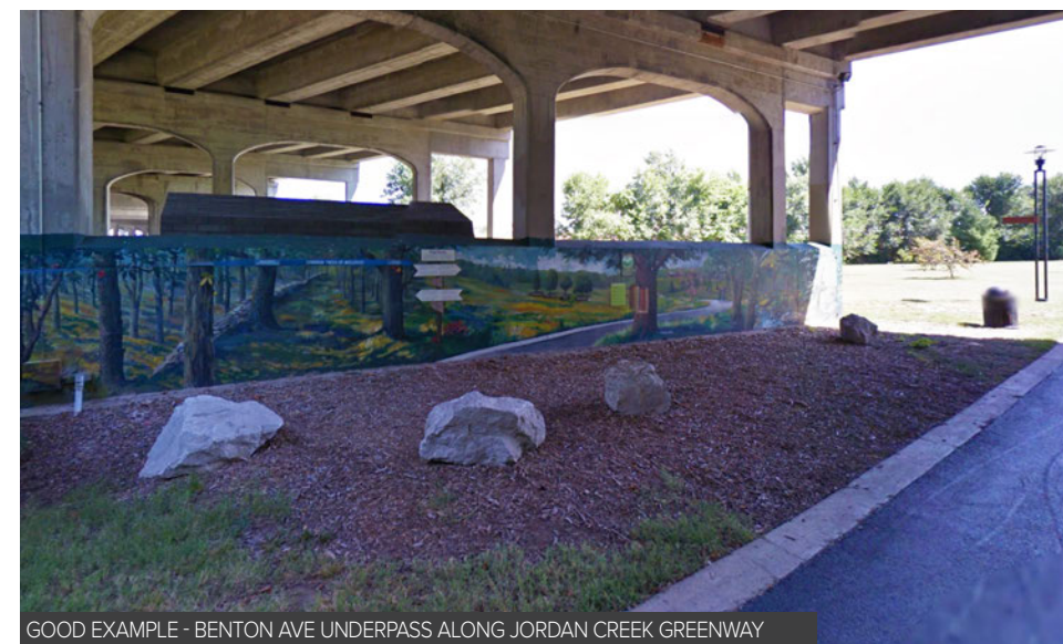
GOOD EXAMPLE - BENTON AVE UNDERPASS ALONG JORDAN CREEK GREENWAY
