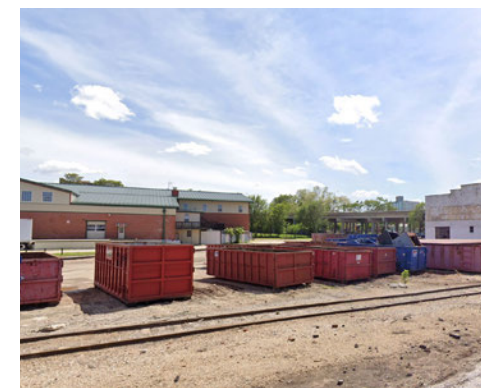
404 JEFFERSON AVENUE EXISTING CONDITIONS
