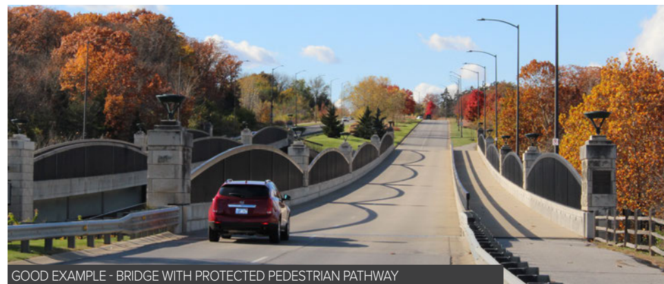
GOOD EXAMPLE - BRIDGE WITH PROTECTED PEDESTRIAN PATHWAY
