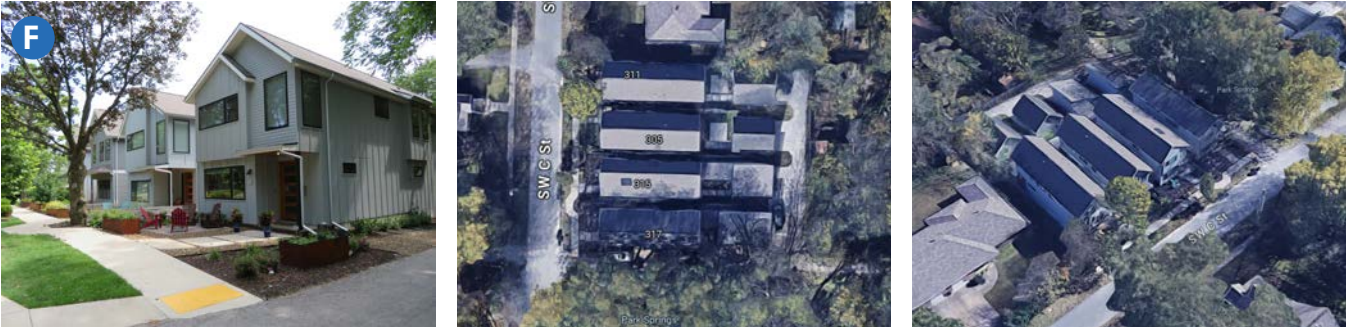
Housing Type: Narrow Lot Single Family Total Housing Units: 4 | Area: 0.48 acres | Density: 8.3 units per acre | Access: Shared Alley
