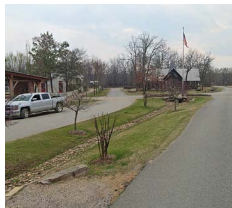
A bioswale in the median directs stormwater towards the lake.
