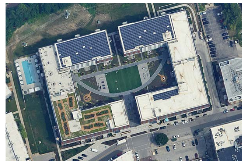
Solar panels on the roof provide on-site energy production.
