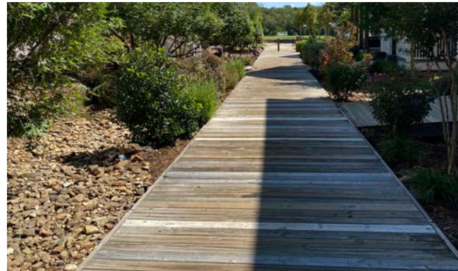
Raised, pervious sidewalks allows stormwater to flow through and underneath.
