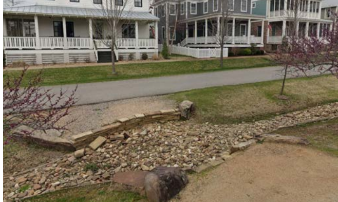
Street-side green infrastructure (bioswale).
