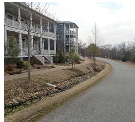
A street-side bioswale directs stormwater away from homes.
