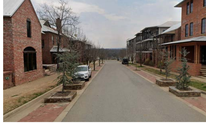
Pervious pavers & tree pits in the parking lane.
