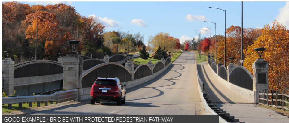
GOOD EXAMPLE - BRIDGE WITH PROTECTED PEDESTRIAN PATHWAY
