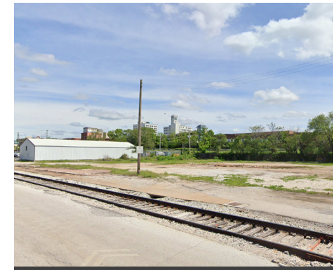
PRIMARY RJC PROJECT SITE EXISTING CONDITIONS
